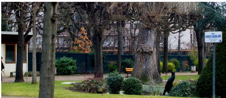
Figure 80: Image of the existing wall
