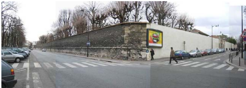
Figure 9: The most imposing part of the external wall – present situation
